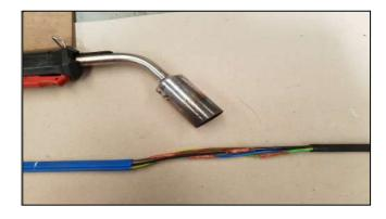
Clean and degrease the previously abraded outer sheaths.
